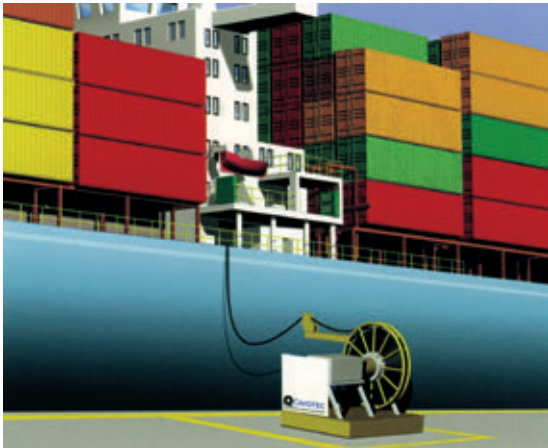
The fixed shore-based power supply
