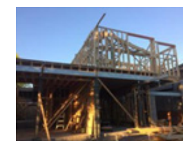
house under construction
