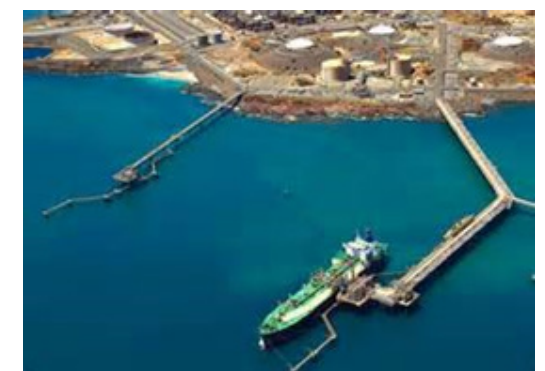
LNG Product Loading Facility
