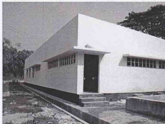
NEW Laundry House (2010)
