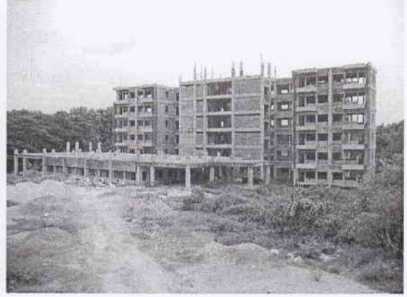
NEW Cadet Block (under-construction) To be completed by Dec 2013
