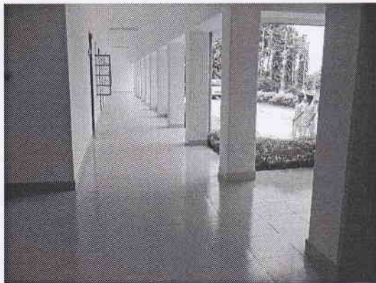
NEW Tiled Corridores in Admin Block (2012)
