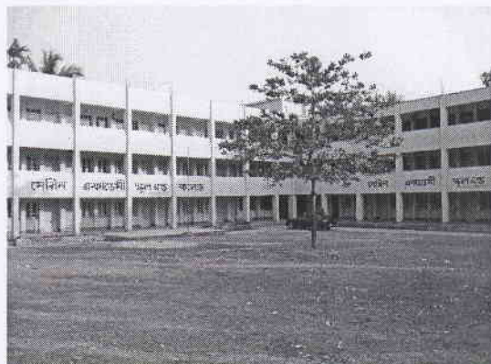
NEW 2 nd Floor of High School (2011)
