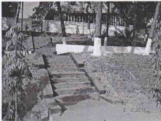
NEW stairway to VIP House (2010)
