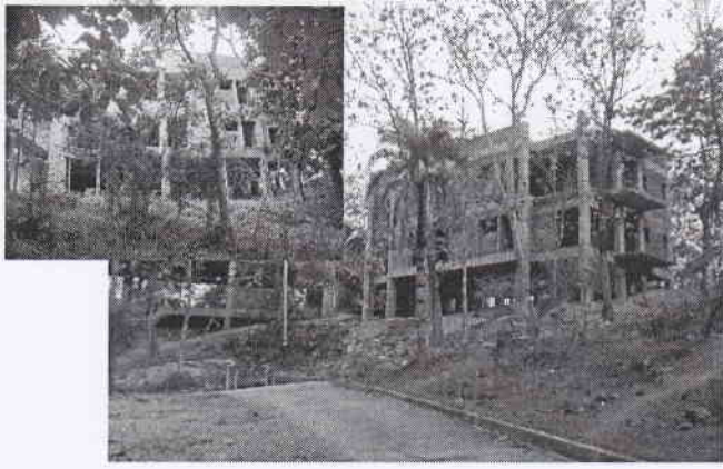
NEW Admin Block (under-construction) To be completed by Dec 2013
